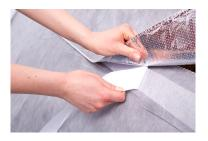
5. Fold the second roll back (100mm), remove the easy peel backing from the double sided tape and secure in place by applying pressure.
