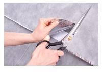
3. Breathe-R can be cut using a craft knife or sharp pair of scissors.
