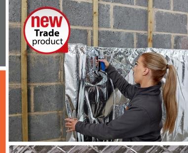
YBS SuperQuilt Trade is a no nonsense high performing multi-foil insulation designed with the Trades person in mind, offering both high thermal properties, along with a highly effective built in vapour control membrane.
