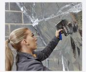
**4.** Tape and seal the perimeter and overlaps using *ThermaSeal* Foil Tape, creating an airtight vapour control barrier.
